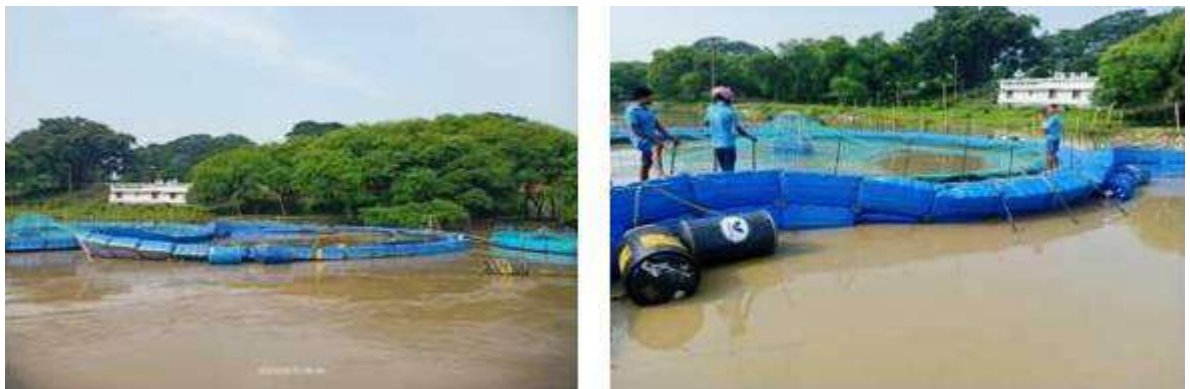
Fig. 333 Cage structure deformed due to water pressure and siltation
