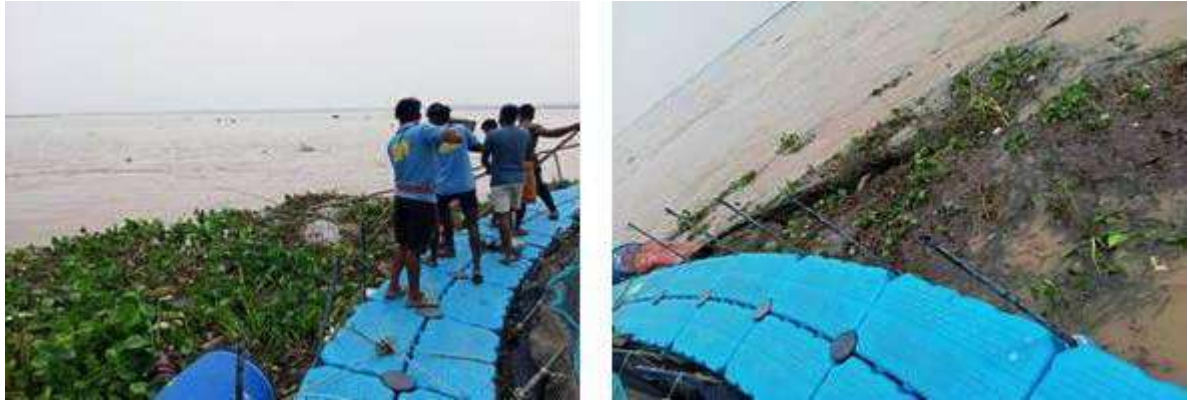
Fig. 332 Macrophytes and other debris clogging the nets
