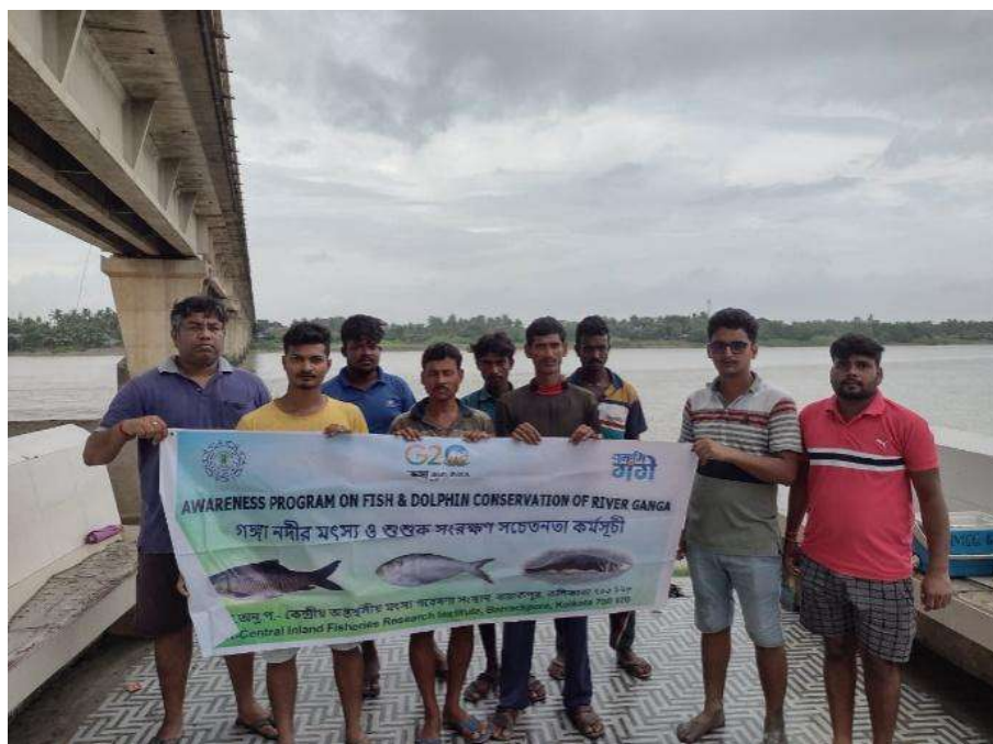
Fig. 255. Awareness at Narghat Rail Bridge in Haldi River (East Midnapur), West Bengal
